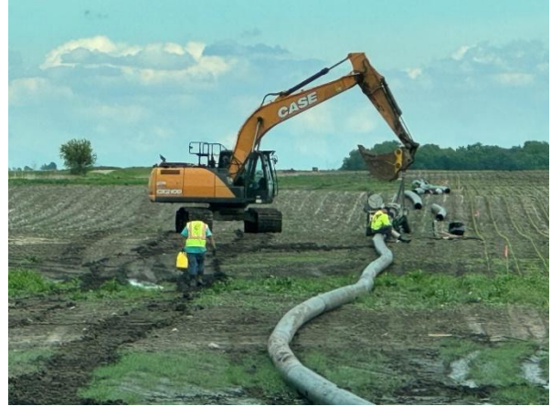
Placing Dewatering Pipe
