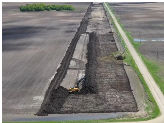
Stripping Topsoil
