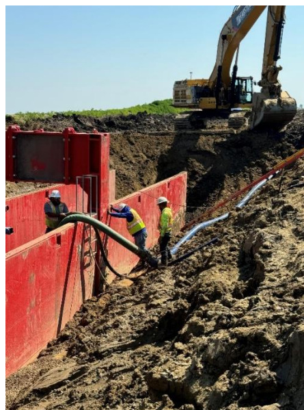
Trench Box w/ Dewatering Pipes
