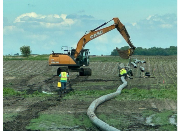
Placing Dewatering Pipe
