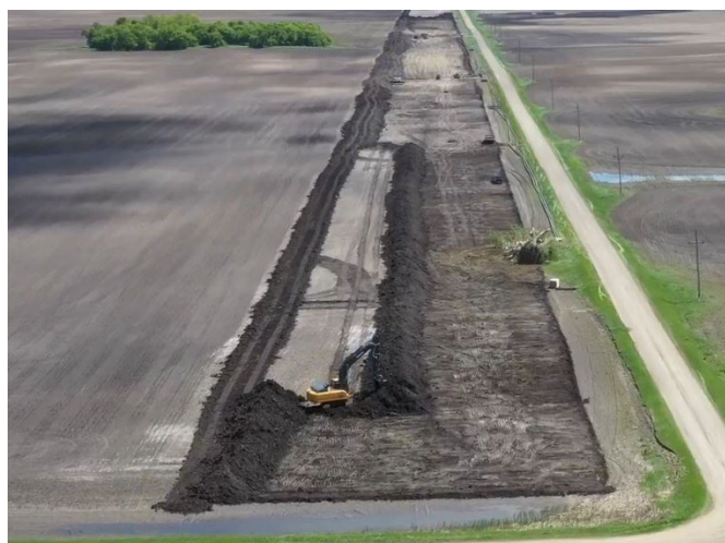
Stripping Topsoil
