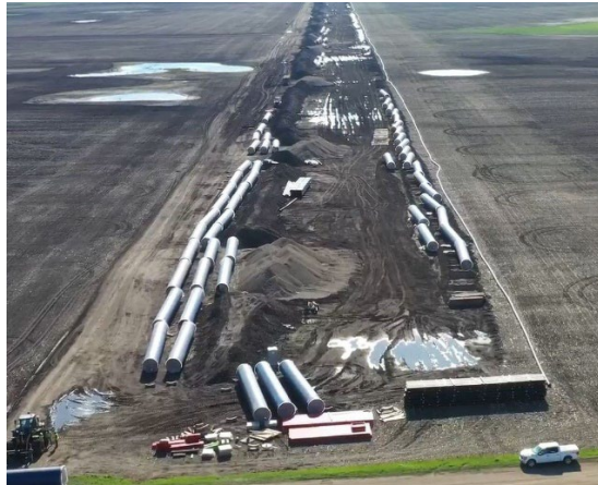
Stored Pipe on Site
