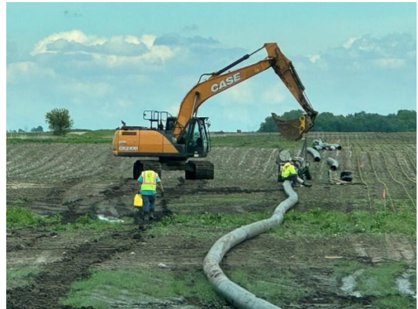
Placing Dewatering Pipe
