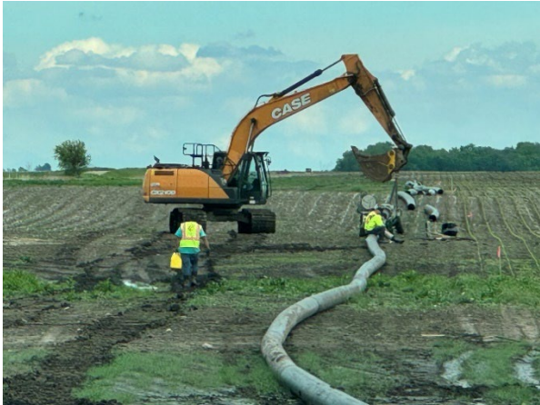
Placing Dewatering Pipe
