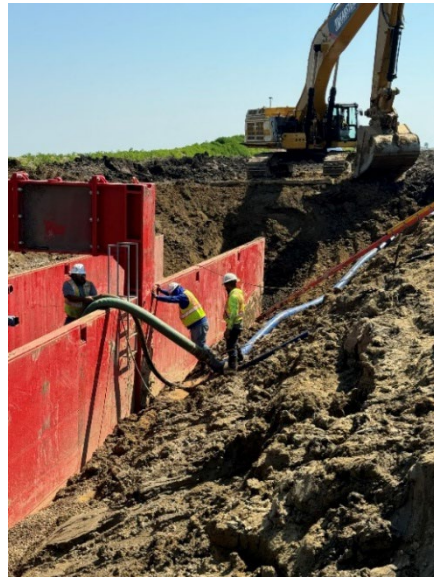
Trench Box w/ Dewatering Pipes
