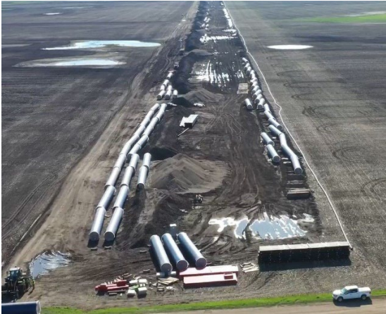
Stored Pipe on Site
