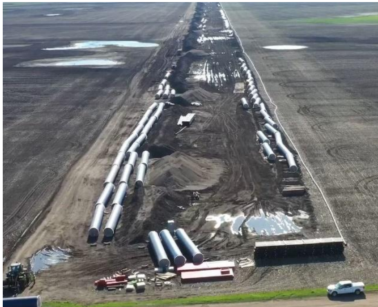
Stored Pipe on Site
