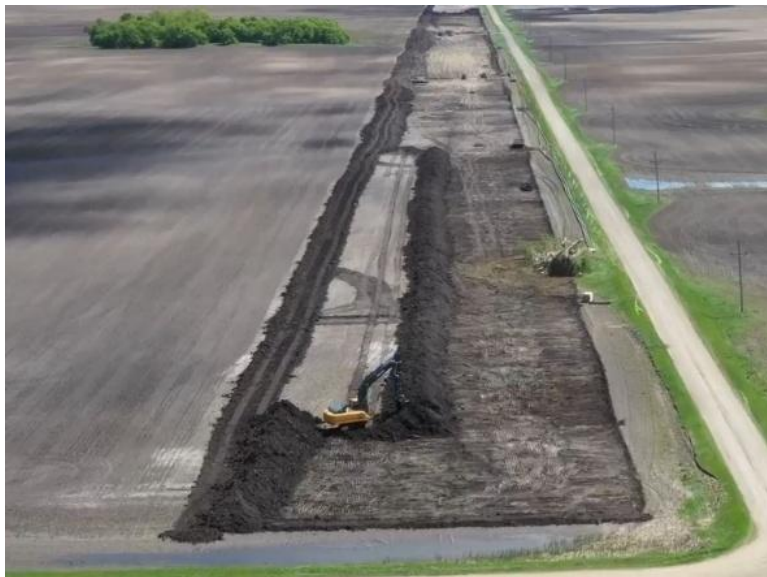
Stripping Topsoil
