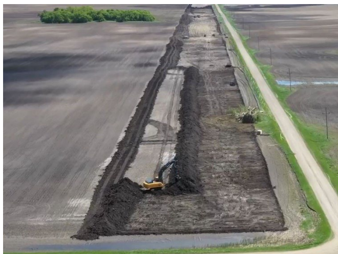
Stripping Topsoil
