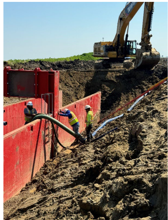
Trench Box w/ Dewatering Pipes
