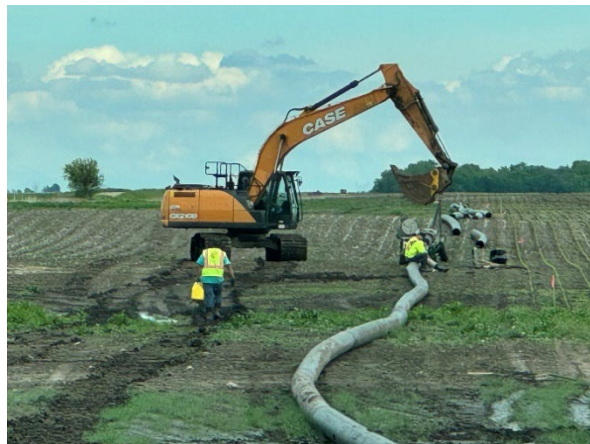
Placing Dewatering Pipe
