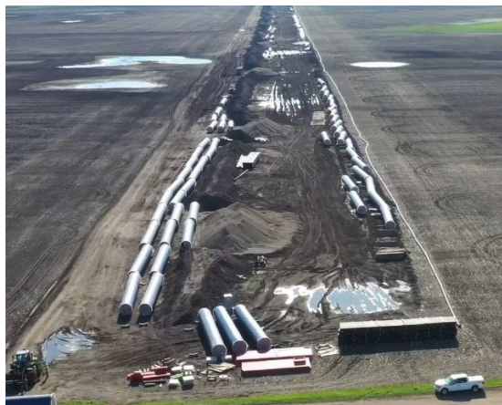
Stored Pipe on Site
