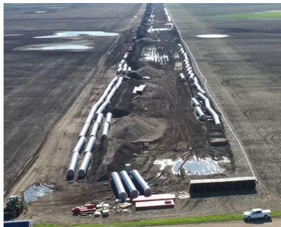
Stored Pipe on Site
