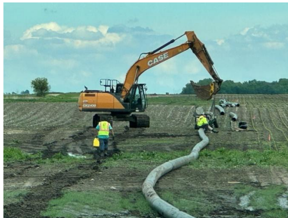
Placing Dewatering Pipe
