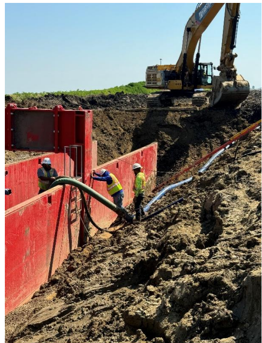
Trench Box w/ Dewatering Pipes
