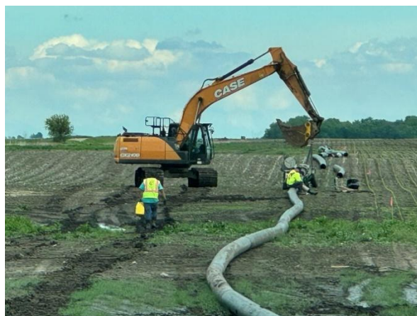
Placing Dewatering Pipe
