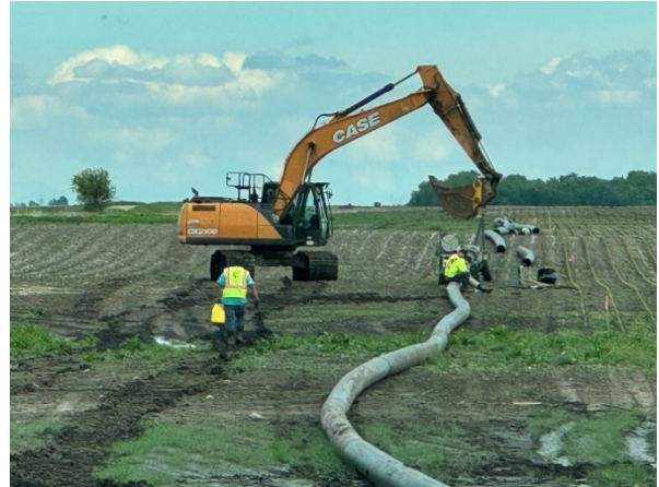
Placing Dewatering Pipe
