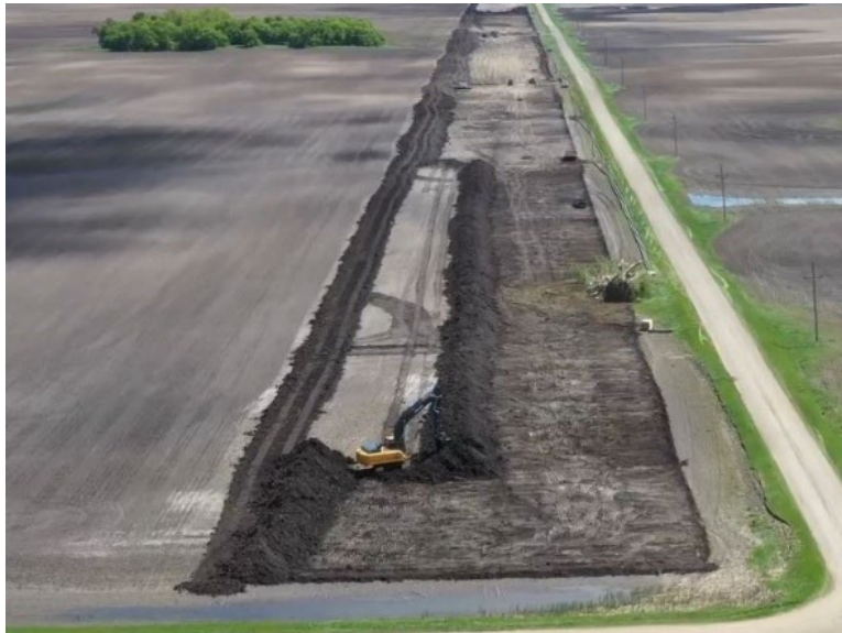
Stripping Topsoil
