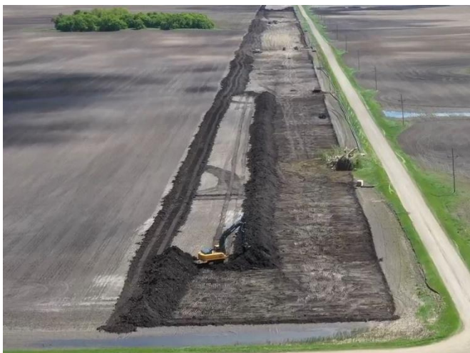
Stripping Topsoil
