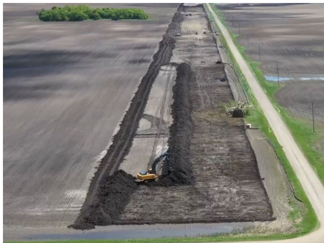
Stripping Topsoil
