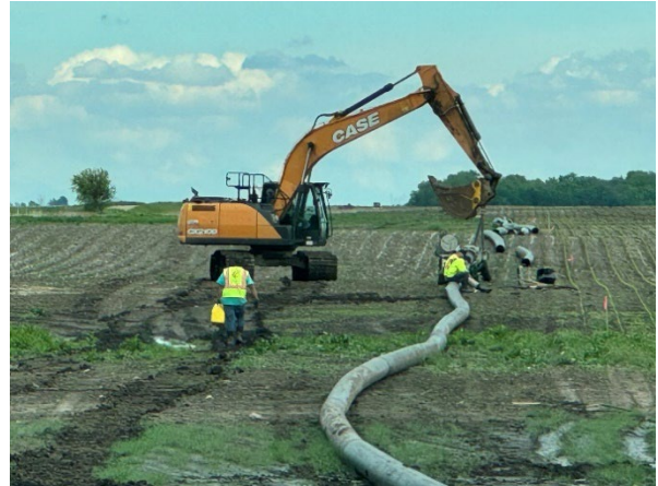
Placing Dewatering Pipe
