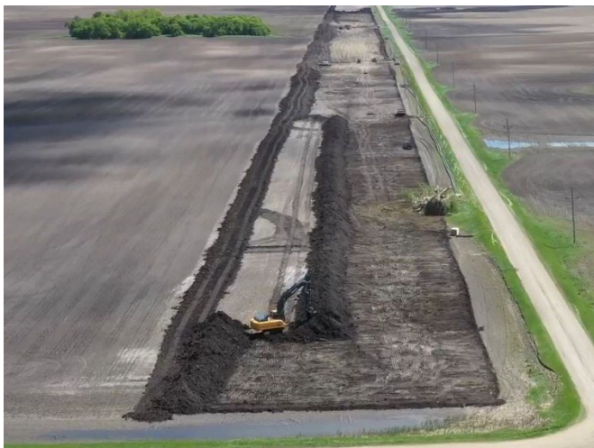
Stripping Topsoil
