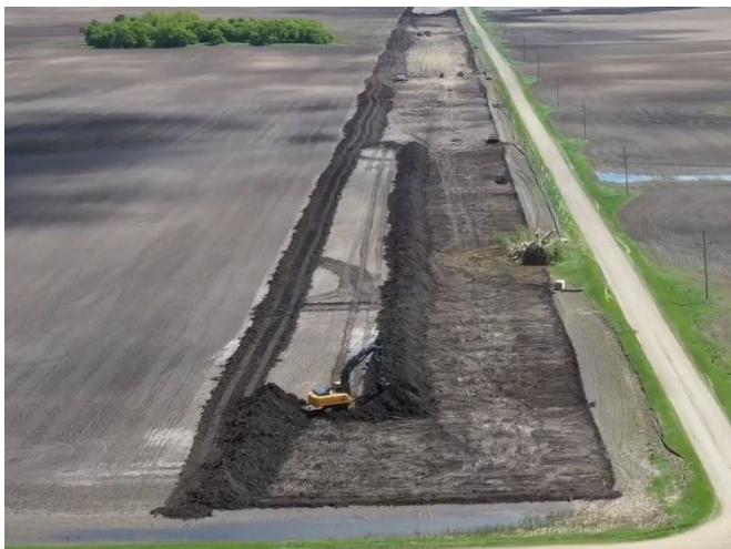
Stripping Topsoil
