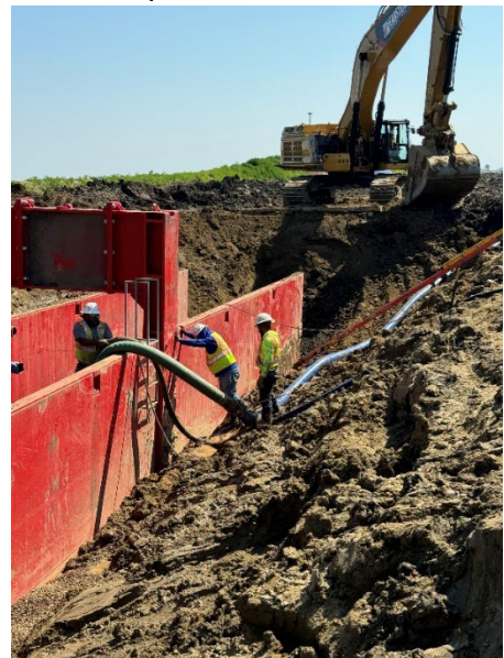
Trench Box w/ Dewatering Pipes
