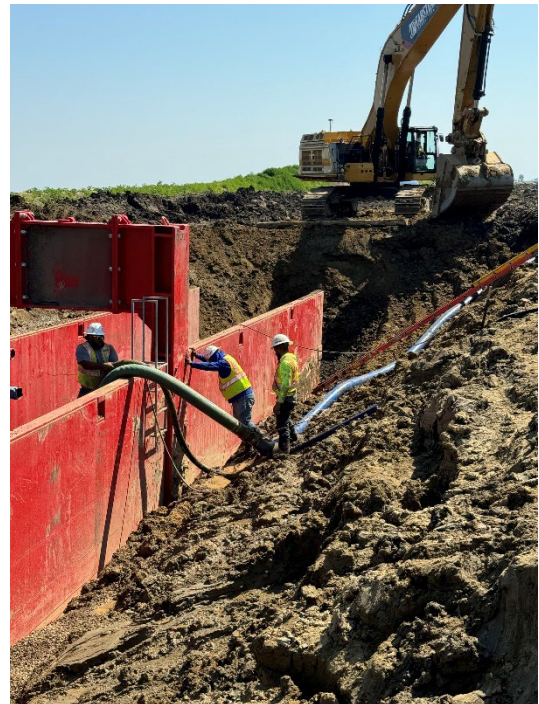
Trench Box w/ Dewatering Pipes
