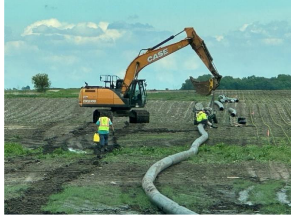
Placing Dewatering Pipe
