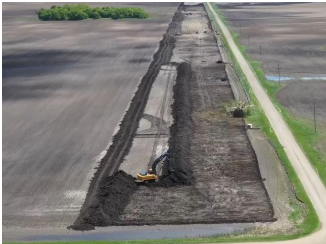
Stripping Topsoil
