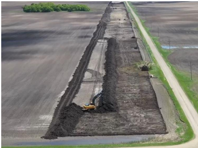
Stripping Topsoil
