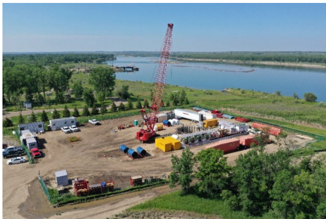
Site Under Construction
