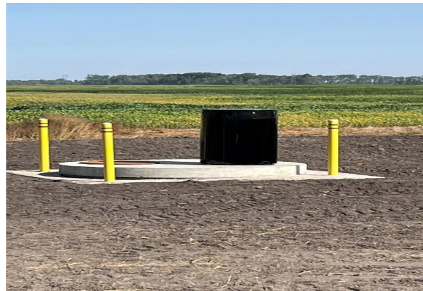
Typical Air Release Manhole
