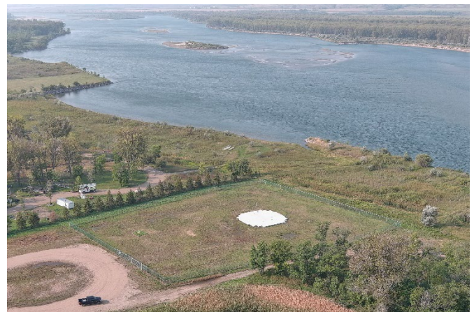
Completed Missouri River Intake
