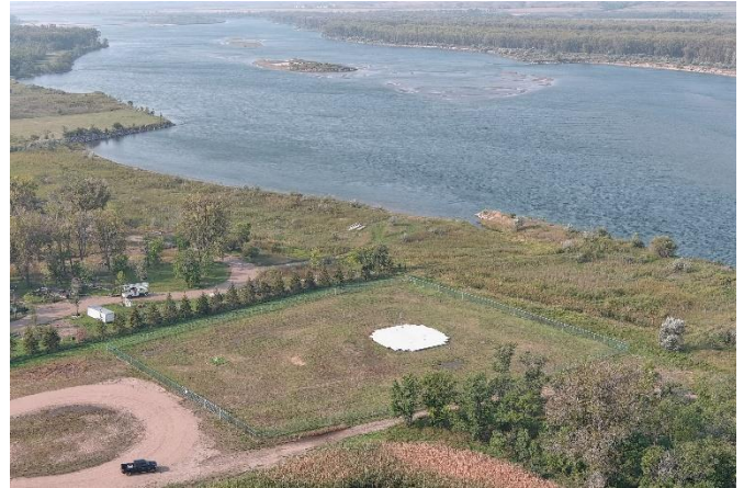
Completed Missouri River Intake
