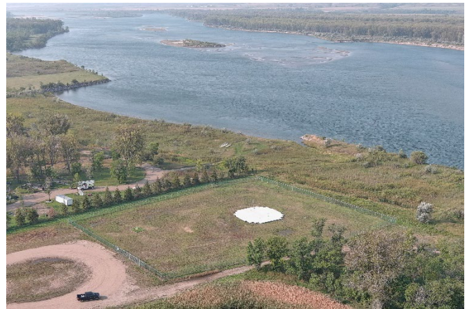
Completed Missouri River Intake
