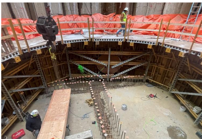
Liner Work on Rebar & Concrete Forms
