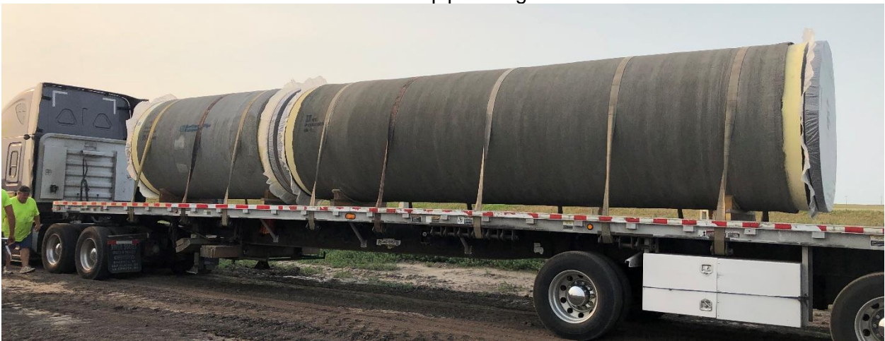
72" carrier tunnel pipe being delivered
