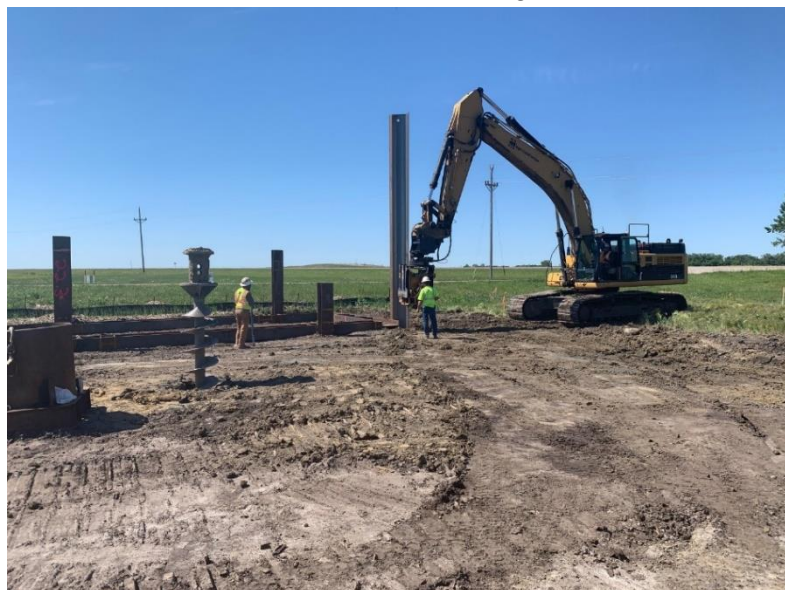
Minger Construction installing the support system for east side tunneling shaft
