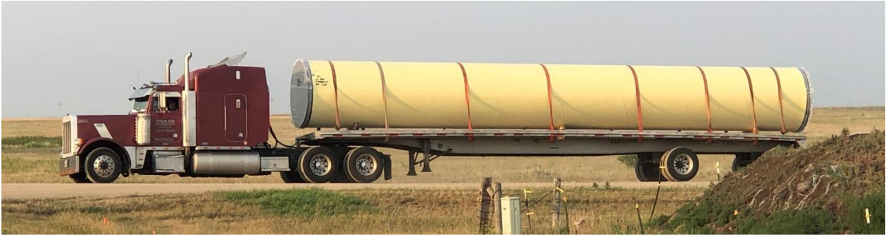
First 72" spiral weld cement mortar lined pipe being delivered
