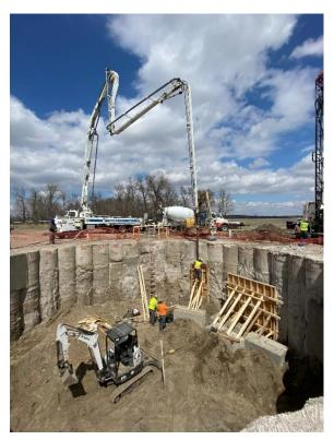
Michels has completed all required secant piles. The dewatering system is installed and waiting for the DEQ discharge permit. Excavating inside the secant structure (wet well) is ongoing currently 25 feet below ground surface.
