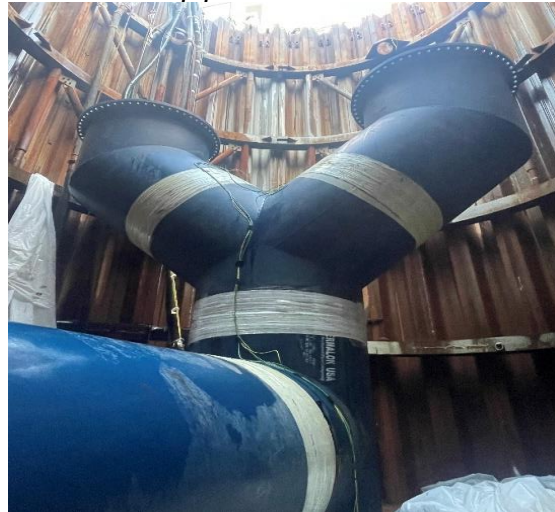
Riser pipe in the coffer dam
