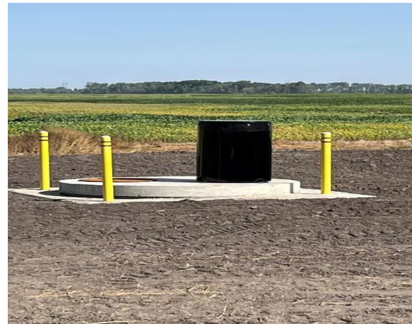
Typical air release manhole
